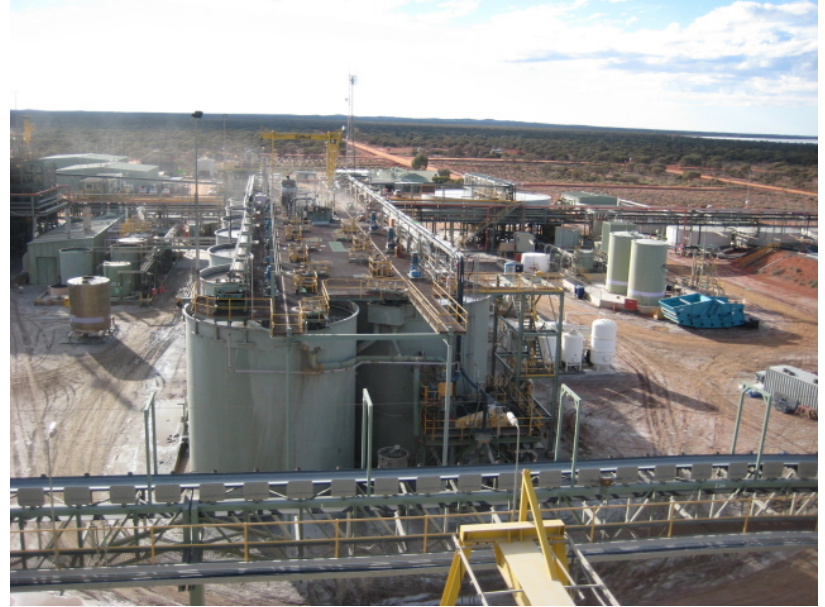
Sunrise Dam Gold Mine (WA) carbon in leach tanks (2009, Wikimedia Creative Commons)
