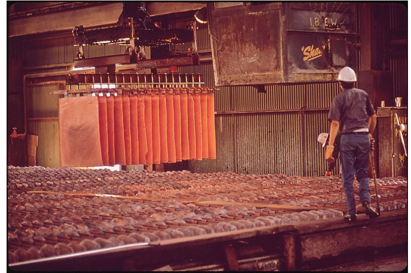
Copper cathodes at the Inspiration Consolidated Copper Company's electrowinning refining plant (Arizona, USA) (CM Keyes 1972, National Archives and Records Administration public domain)
