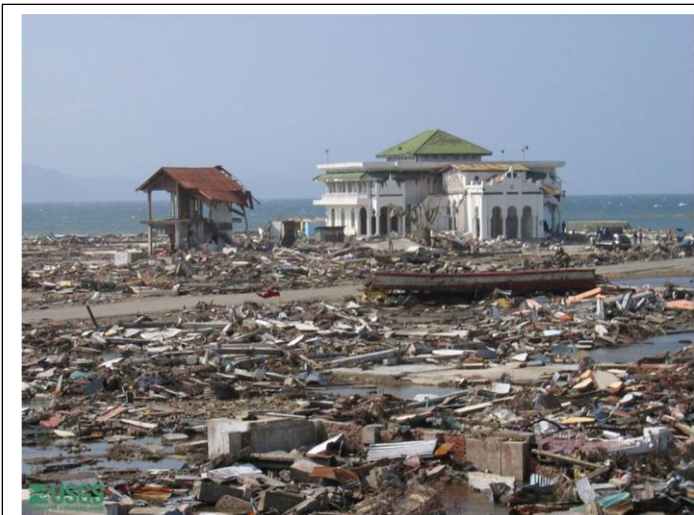
Figure 2. A mosque is left standing in the rubble of Banda Aceh after the Boxing Day tsunami in 2004. Mosques often have an open ground floor this helped it withstand waves that reached the middle of the second floor. (USGS 2005, public domain)
