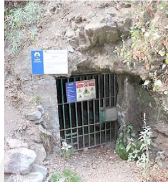
Shaft entry blocked for safety at Barranco de Badajoz mine in Tenerife (2019, Wikimedia Creative Commons)
