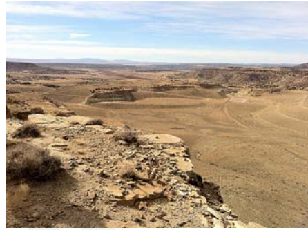
The former Jackpile-Paguate uranium Mine in New Mexico USA has been backfilled and contoured. (M Gant, National Institute of Environmental Health Sciences 2013, Public Domain)
