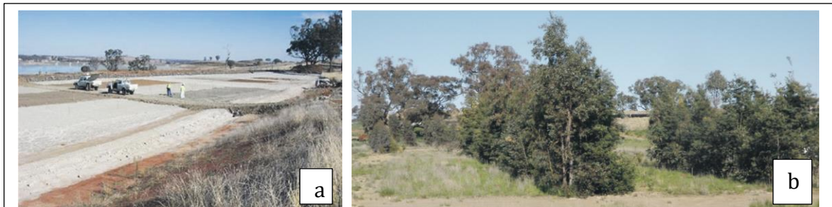
Figure 3: Tailings revegetation trials. (a) Construction of plots for rehabilitation in 2004. (b) Significant growth of vegetation seen in 2010, despite drought. (provided by Newcrest Mining Ltd)
