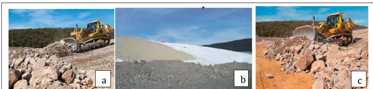
Figure 2 (a) waste piles are contoured to less than a 18° slope, (b) HDPE and compacted clay layers seal the waste, and (c) inert rock and soil are placed on top of compacted clay (from Cadia District Heritage & Recreational Area Guide Book)
