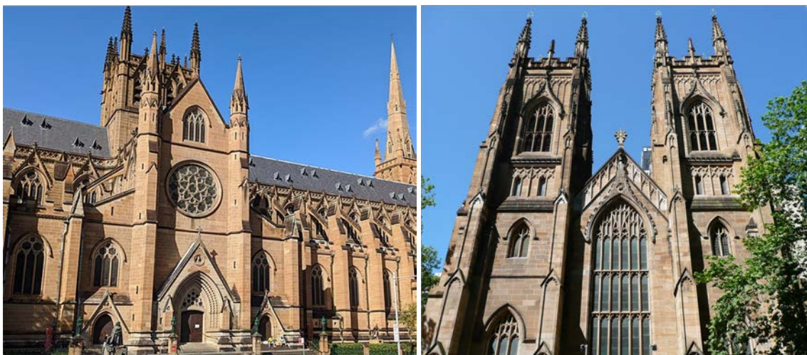
St Mary's Cathedral (left) is built of yellow block sandstone. St Andrew's Cathedral (right) is built of quartz-rich sandstone. (St Mary's by MDRX 2020, St Andrews by Hermione9753 2010, Creative Commons)
