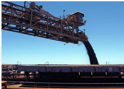
Rio Tinto iron ore shiploader in the Pilbara (C Hargrave, CSIRO Science Image)
