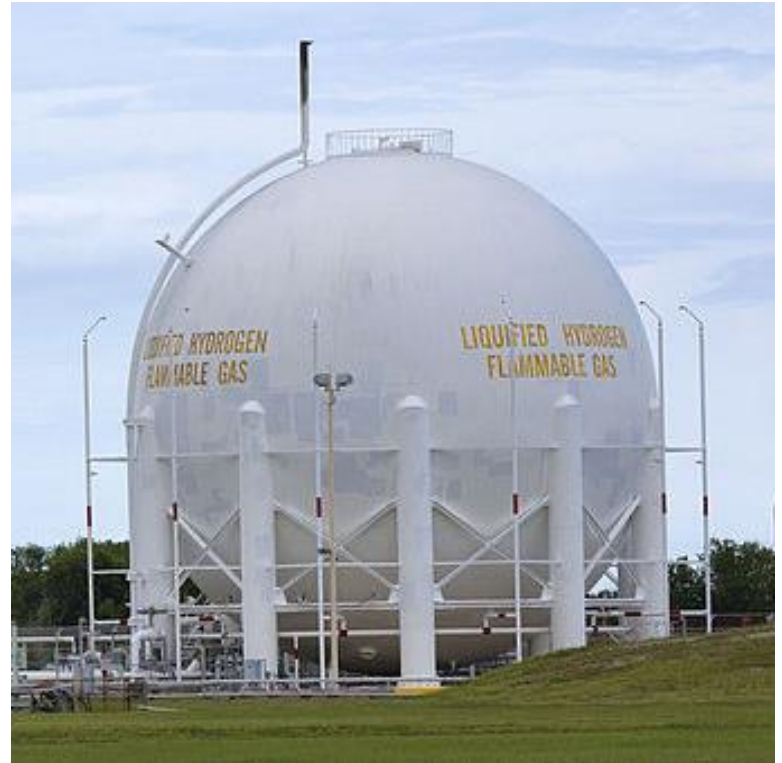
Liquid hydrogen storage tank at Kennedy Space Center was used to fuel the space shuttle. (TomFawls 2013, creative Commons 3.0)
