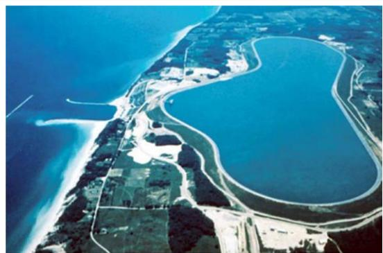
A pumped hydroelectric storage facility in Michigan (USA) is used to store energy from the electricity grid and release it as needed. (US Government 2011, public domain)
