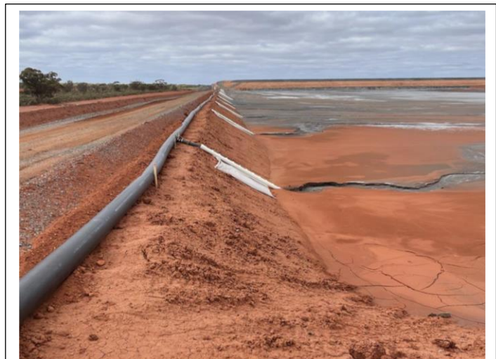
Tailings being pumped into a tailings storage facility at Mungari (courtesy of Evolution Mining)
