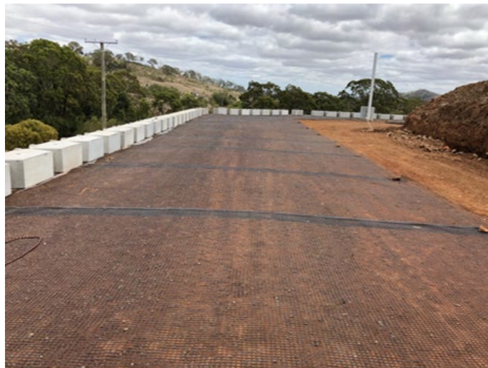
Figure 2: A geogrid or mesh laid over the dirt to reinforce the soil and stabilise the ground.
