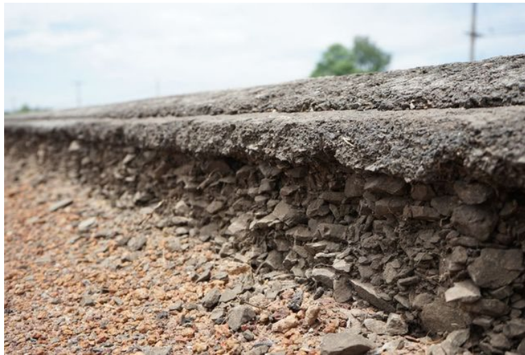
Figure 8: Road base (source: https://www.bracingsystems.com/what-is-road-base-and-why-does-it-matter )
